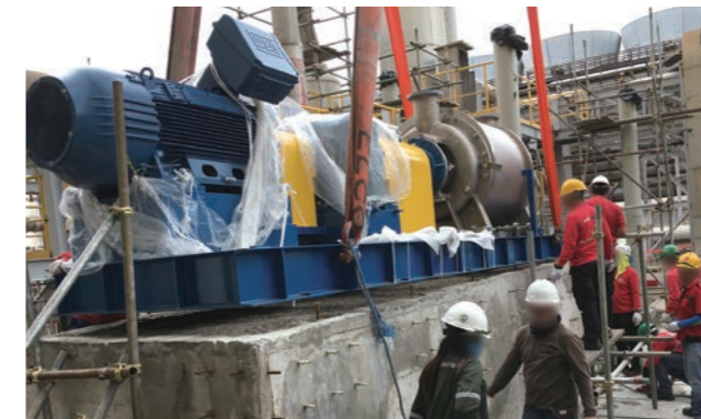
Installation instruction for large liquid ring vacuum pump 大型真空ポンプ据付指導
